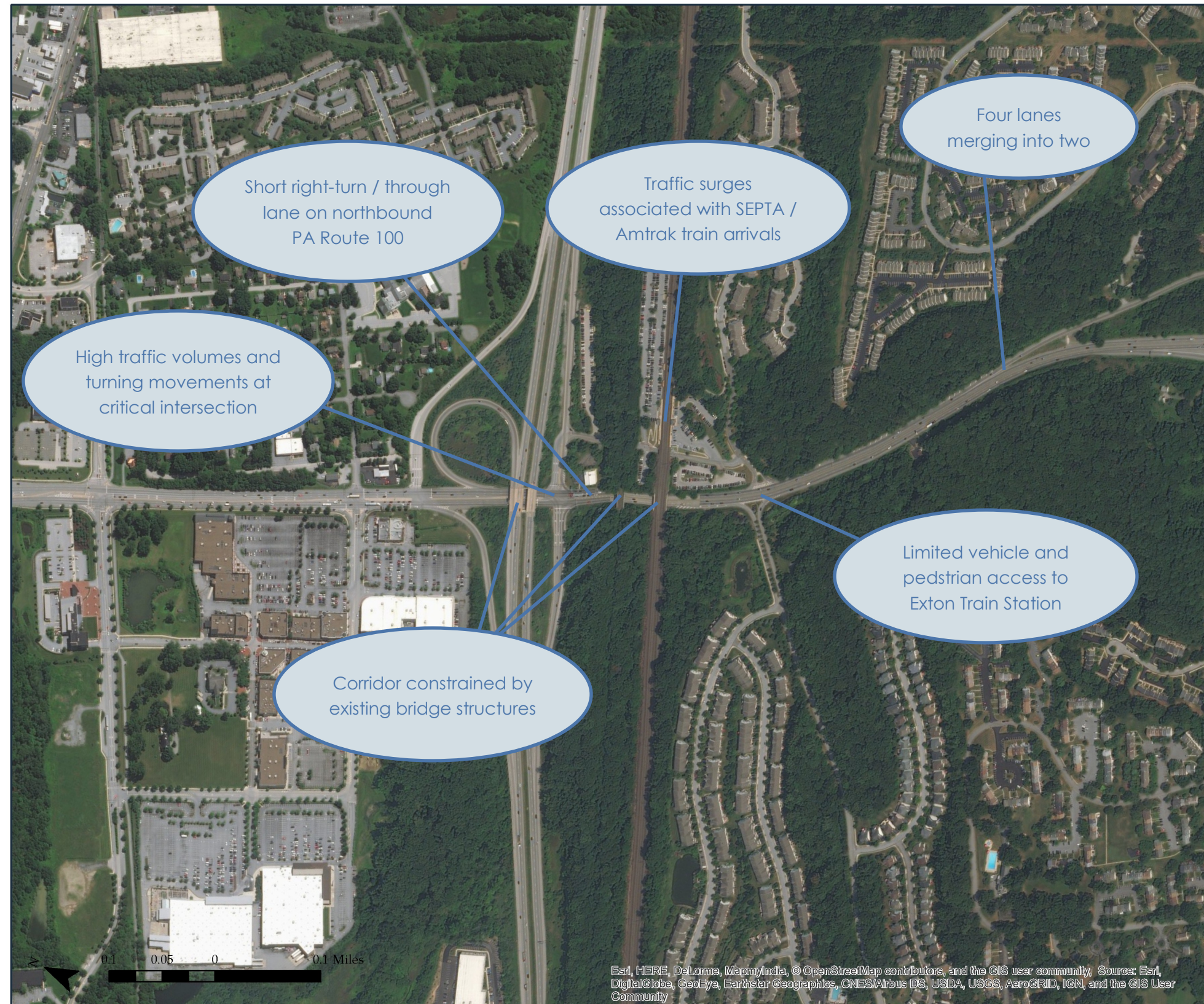
Figure 2.5: Key Existing Conditions Findings
