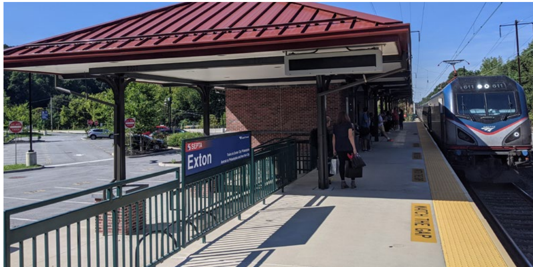
Completed in 2020, the rebuilt Exton station incorporates full ADA-access, high-level boarding platforms, a station building, and additional train shelters.
