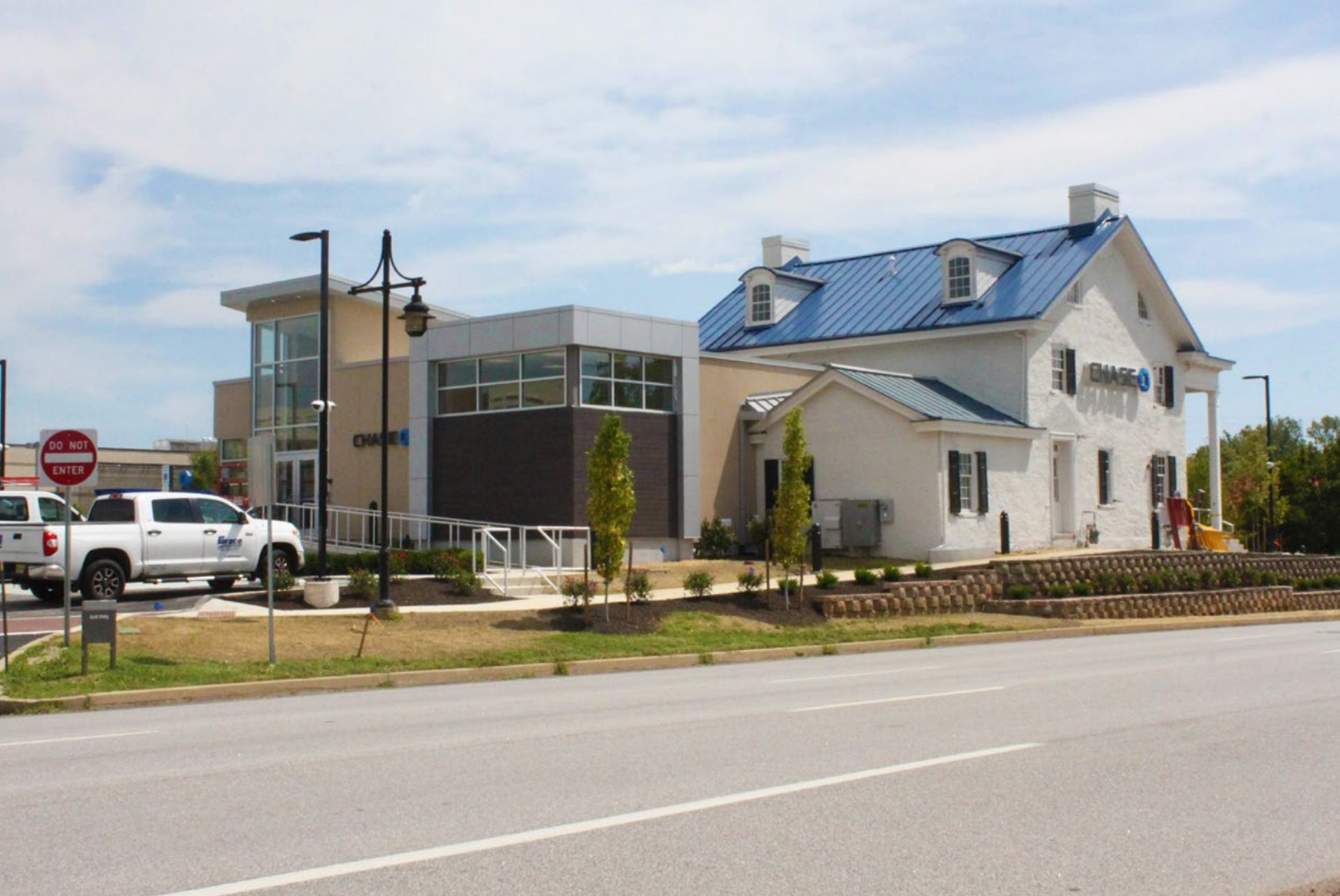
Adaptation and reuse of historic properties such as the former Malvern Federal Bank building (now a Chase Bank) provide for a glimpse into the tapestry of history in the Township for residents and visitors alike.
