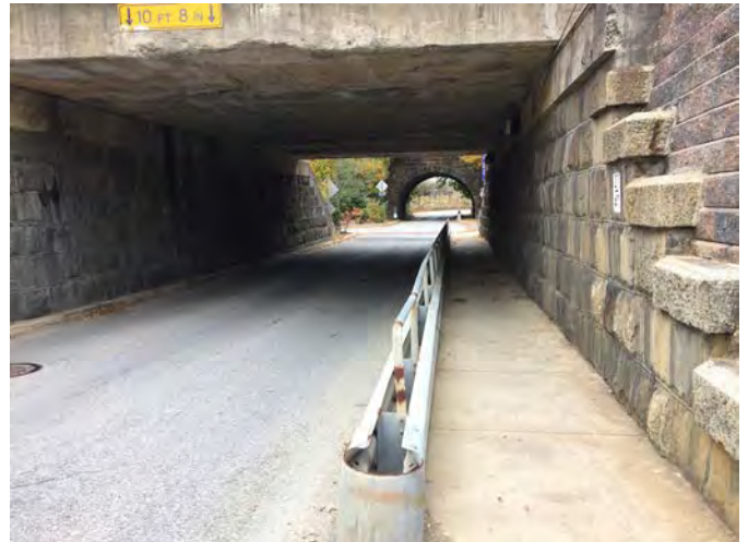
SEPTA rail right-of-way underpass within station area.
