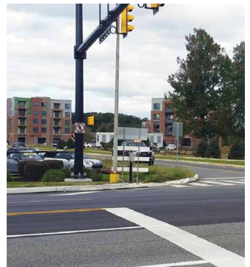
The new Keva Dr. and traffic signal at Lincoln Hwy. Keva Dr. connects Lincoln Hwy. to Waterloo Blvd., alleviating traffic at the intersection of Whitford Rd. and Lincoln Hwy.
