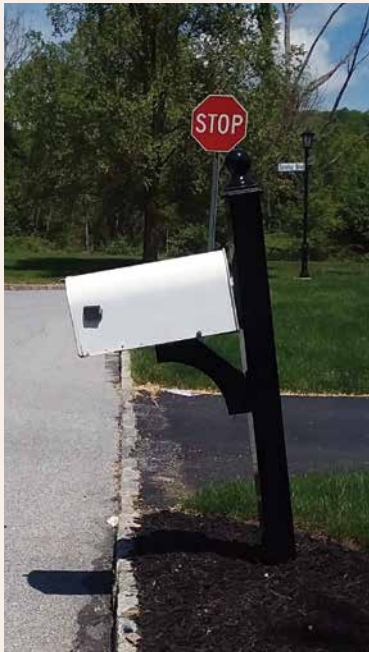
Leaning mailbox that needs to be straightened.
