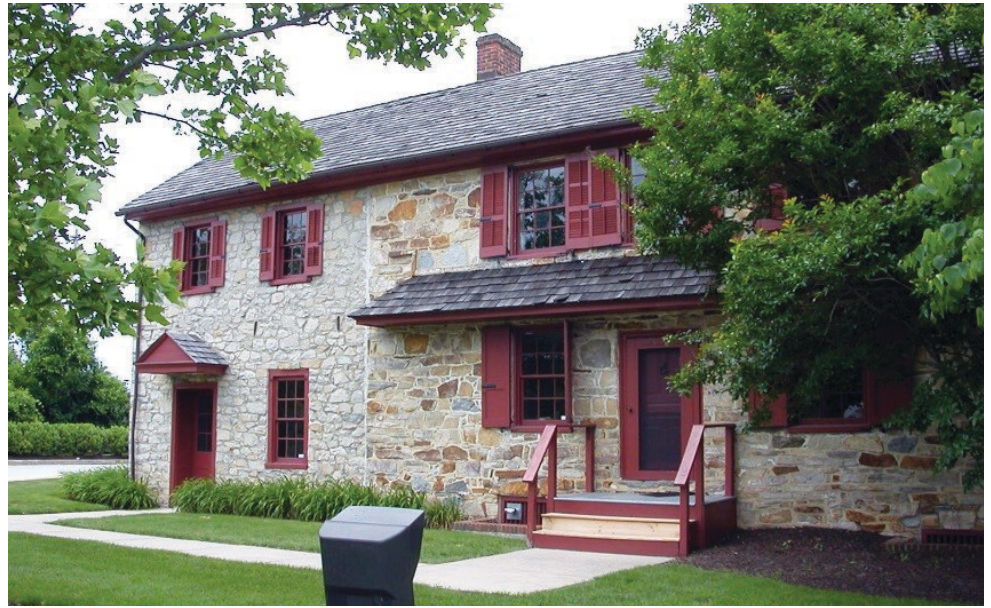
The original Historical Commission conducted business in the Zook house on the Exton Mall grounds.
