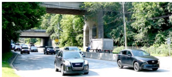
A third northbound lane is proposed to extend from Pottstown Pike to the US Route 30 Bypass. This will help alleviate congestion with additional capacity approaching the Town Center.
